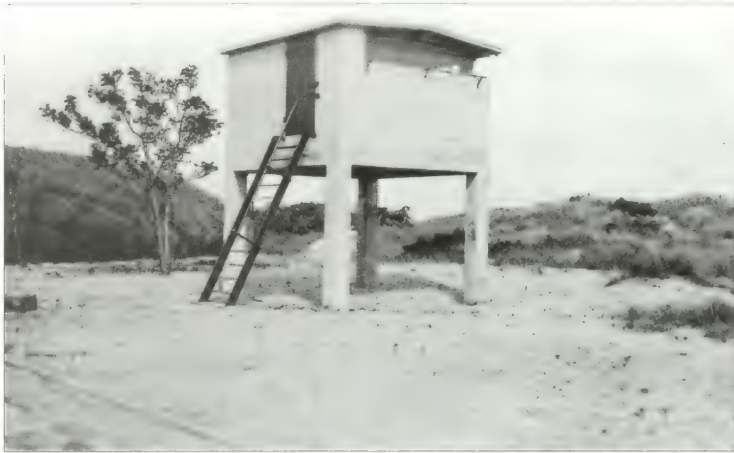
Figure 2.86. View looking northwest at coincidence range finder station east of Battery Morris, circa 1921. The instrument height of the range finder and the area north of the station free of large, woody vegetation combined to provide unimpeded views of the water and improved fire control for Battery Morris (GATE 7893).
